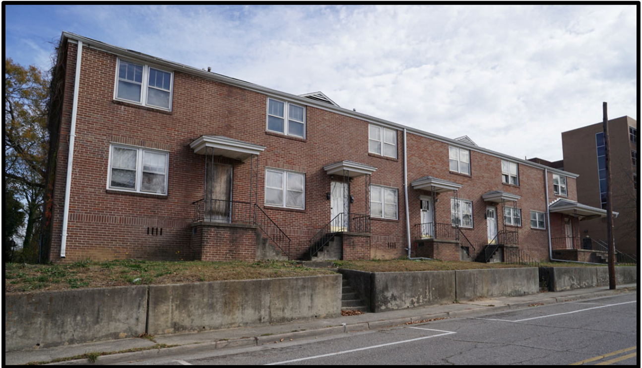
Photo 14 – vacant apartments across Oak Street from the site
