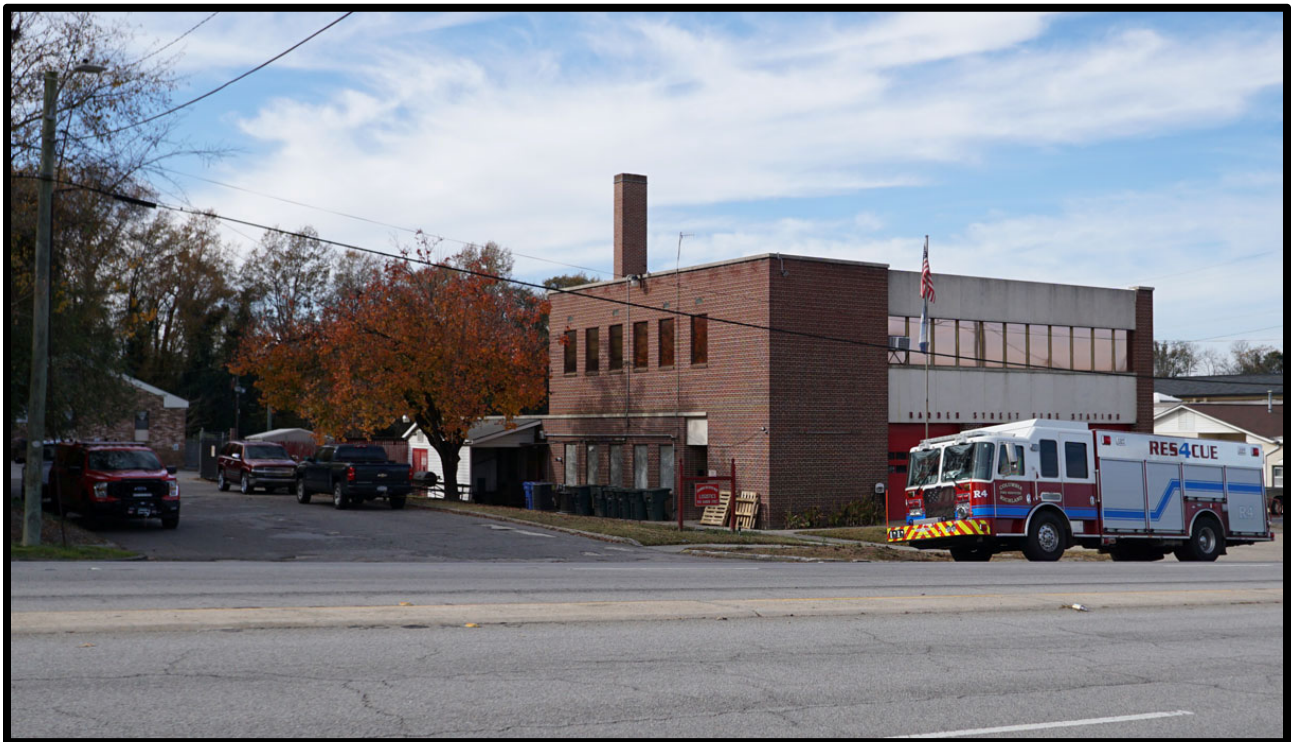
Photo 10 – Columbia Fire Department Logistics across Harden Street from the site
